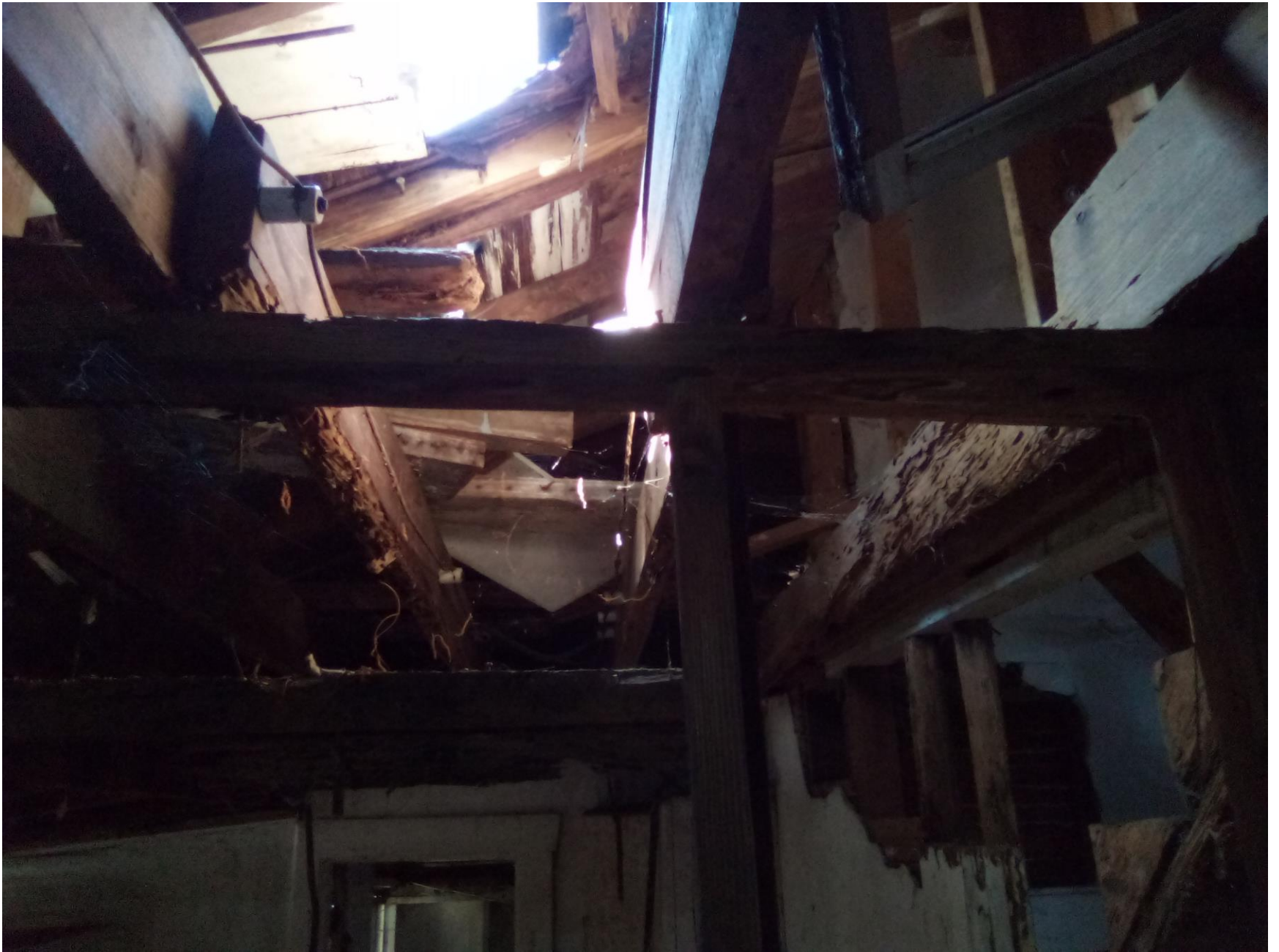
Trusses and hole in Roof
