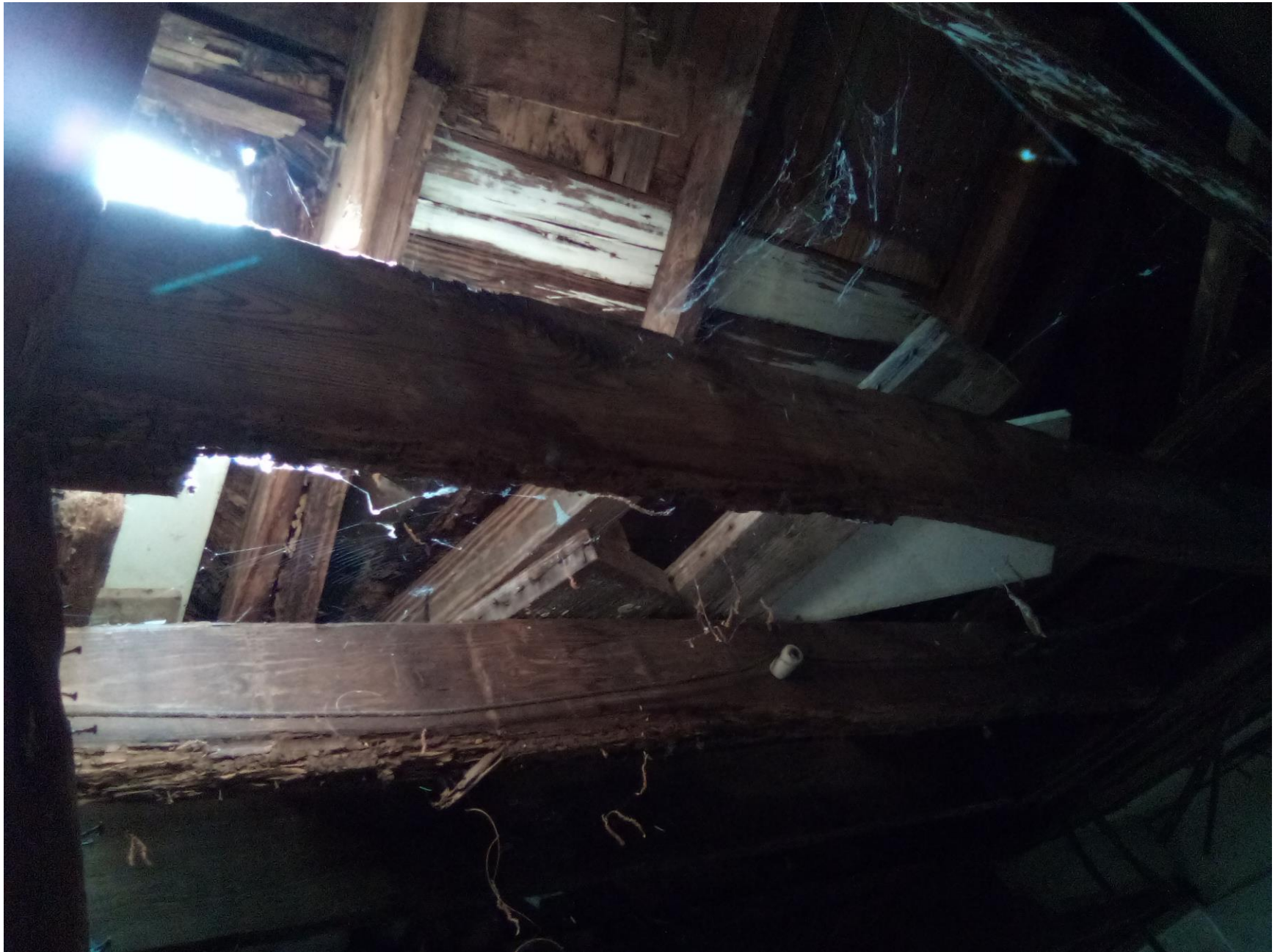
Trusses and hole in Roof
